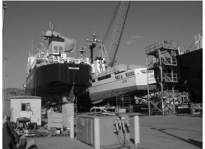
The new dry dock at Curtis Bay lifts the cutters out of the water so that they can move around on dollies.
